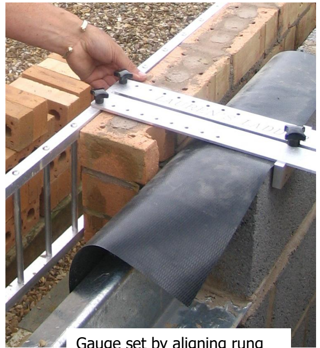
Securing ladder sections
