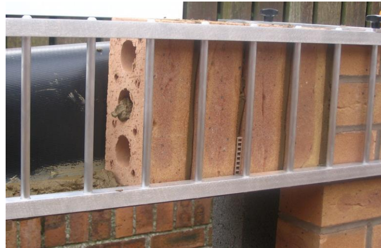
Courses are laid more quickly and accurately, and Laurens Ladder holds them in place until set.
