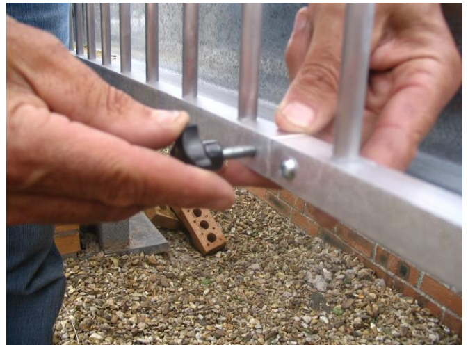
Securing ladder sections
