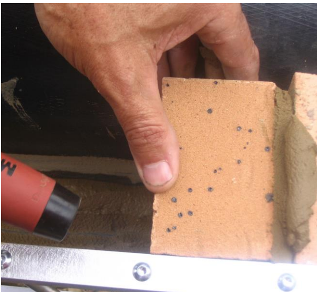
Each brick is laid behind Laurens Ladder using the top bar as a level and the vertical bar as a mortar joint gauge.
