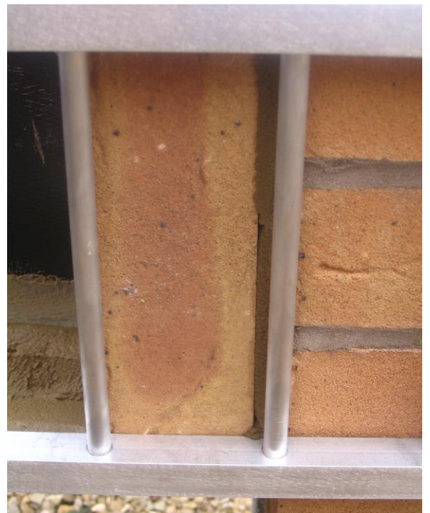
Top and bottom bars hold each brick in place.
