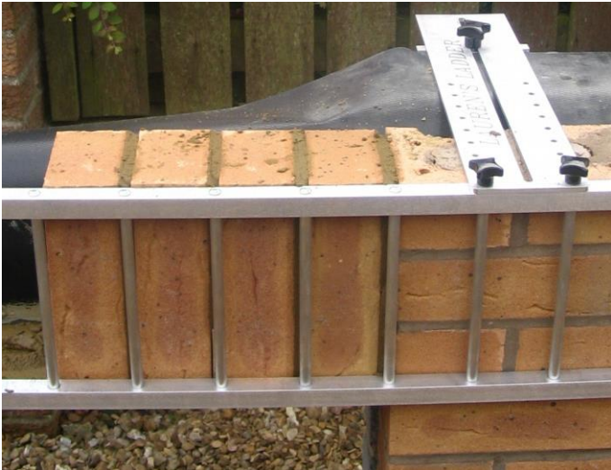
Courses are laid more quickly and accurately, and Laurens Ladder holds them in place until set.
