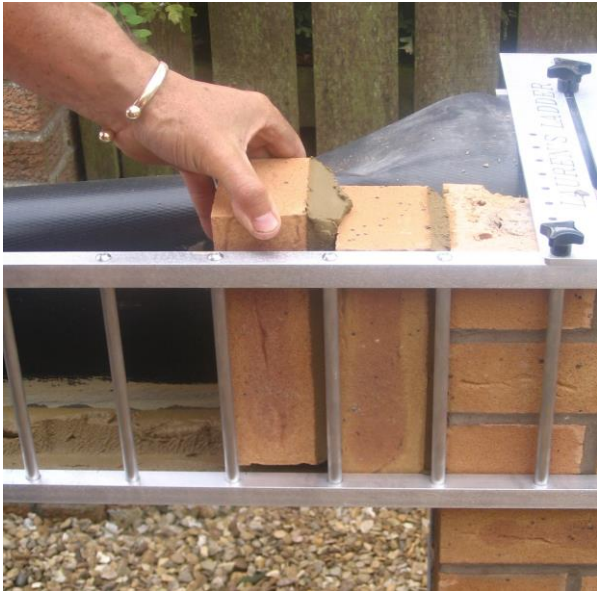
Each course accurately positioned and held in place.
