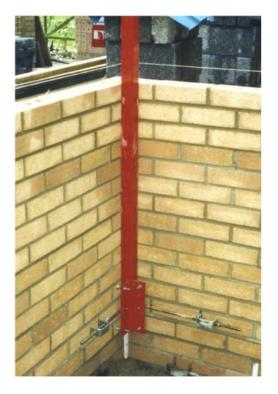
Screw the M12 wing nut onto the clamping bolt (wings first) and engage the hooked end of the bolt into the hole in the Profile side plate.
