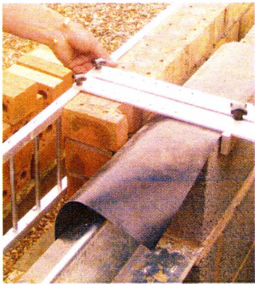
Gauge set by aligning rung
