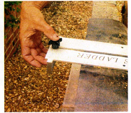
Clamps adjustable for cavity width
